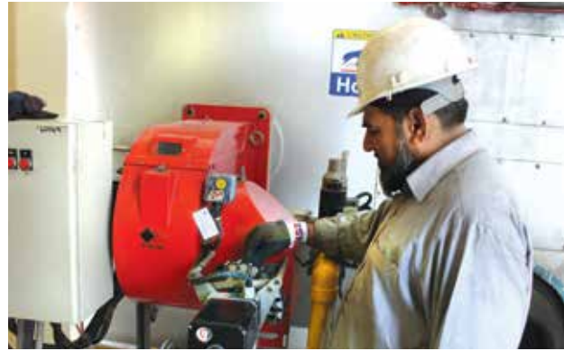
The Chemicals team executes its annual plant shutdown
