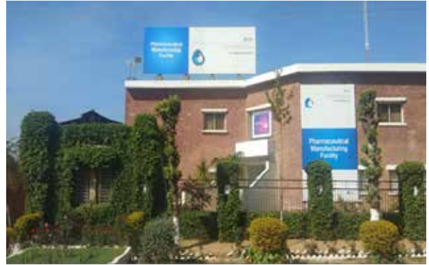
A view of the Cirin Plant at Hattar
