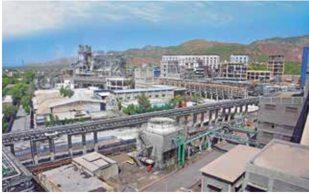
The Phase 2 of 150,000 tonnes per annum Light Ash capacity expansion at the Soda Ash Plant, being expansion of 75,000 tonnes per annum, is now underway
